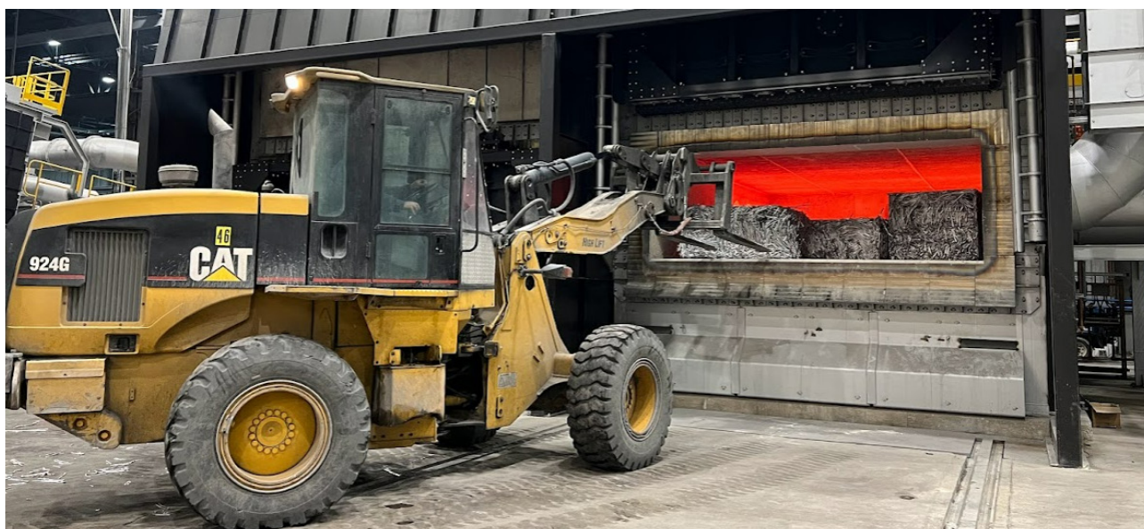
The first recycled aluminium being remelted in the new recycling and casting center in Huntingdon, Gränges Americas.
