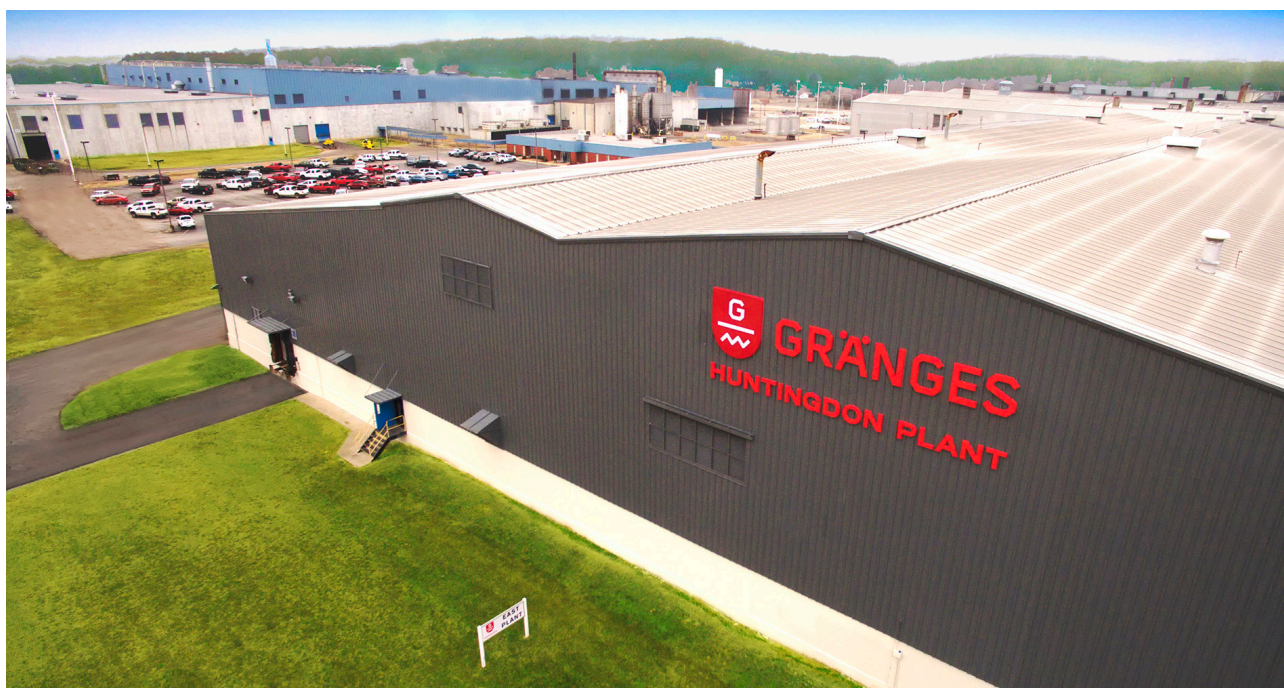
Gränges production facility in Huntingdon, Tennessee, USA.
