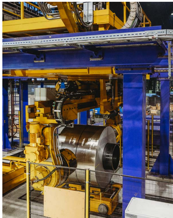
Production started in the new cold-rolling mill in Konin in the first quarter.
